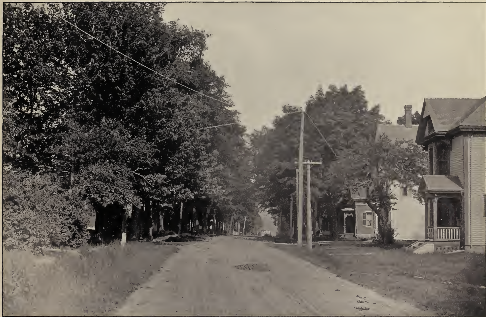
HIGHLAND AVENUE, LOOKING DOWN FROM AUTUMN STREET.
